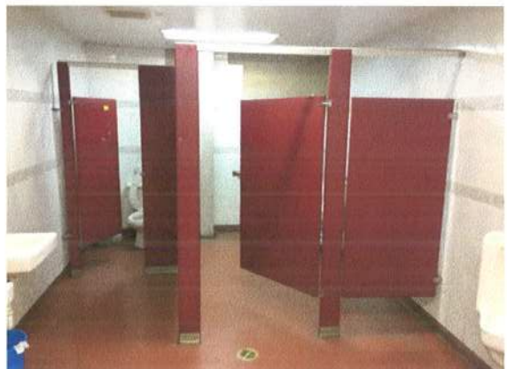
Retail area bathroom (Photo Taken on June 16, 2015)
