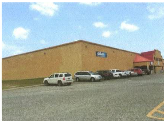
Front and side exterior (Photo Taken on June 16, 2015)
