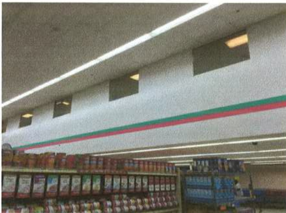
View of upper level office area (Photo Taken on June 16, 2015)
