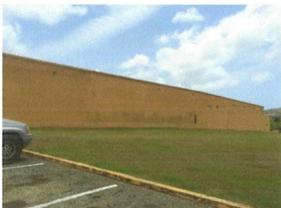
Side exterior (Photo Taken on June 16, 2015)
